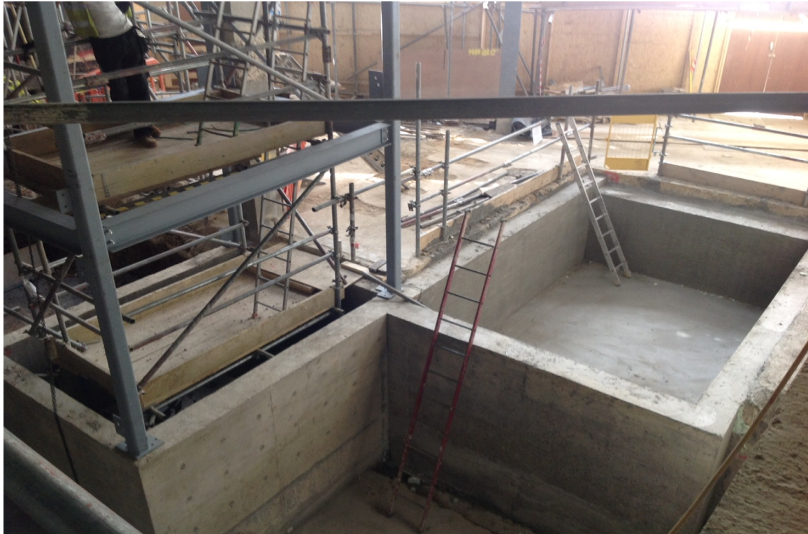
Formation of New Escalator Pits
