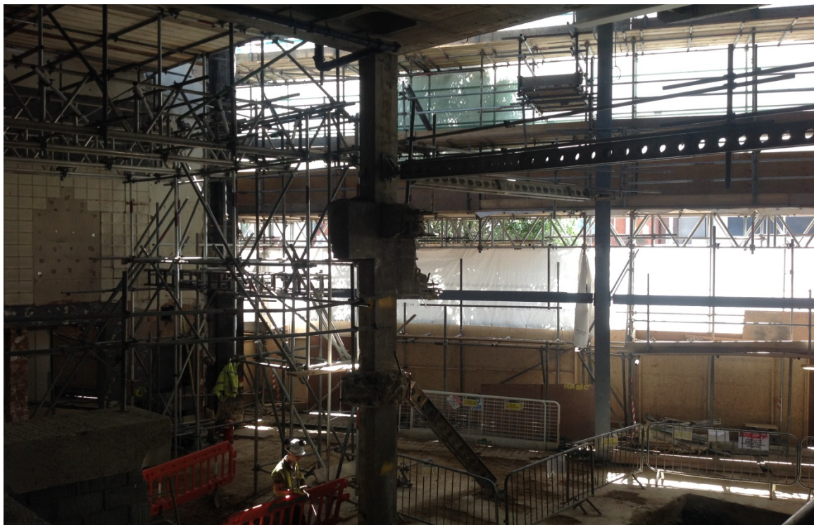
Construction of New Shopping Centre Entrance
